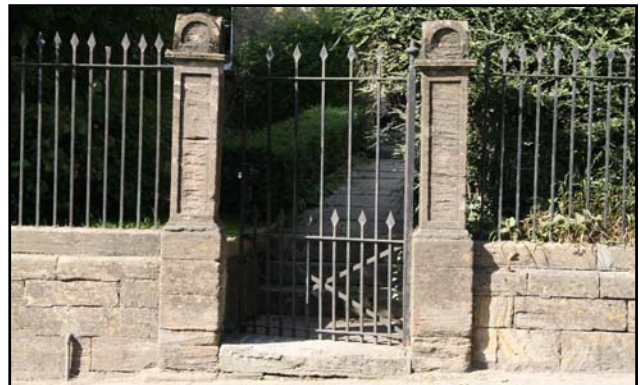
Walls, gate piers and ironwork, North Street
