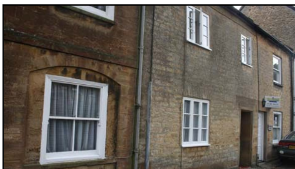
Varied windows, sash, casements and marginally-glazed sash, Oxen Road
