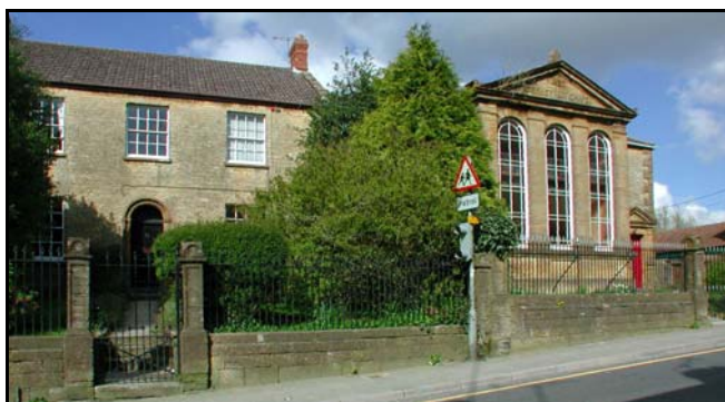
Former Baptist Church and manse, North Street
