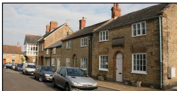
Key unlisted buildings, Court Barton
