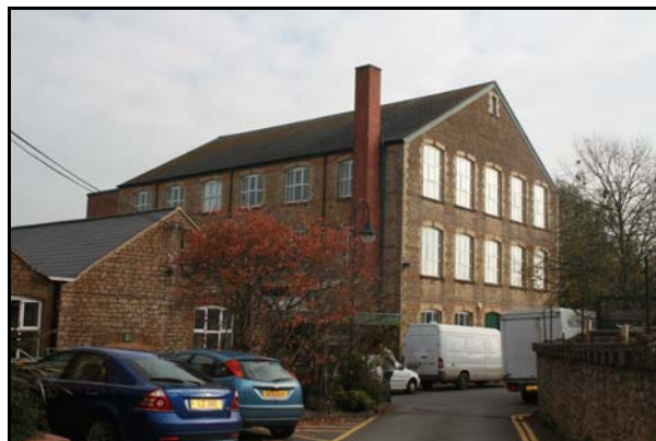
Former Robert Bird & Co. webbing and weaving factory, South Street
