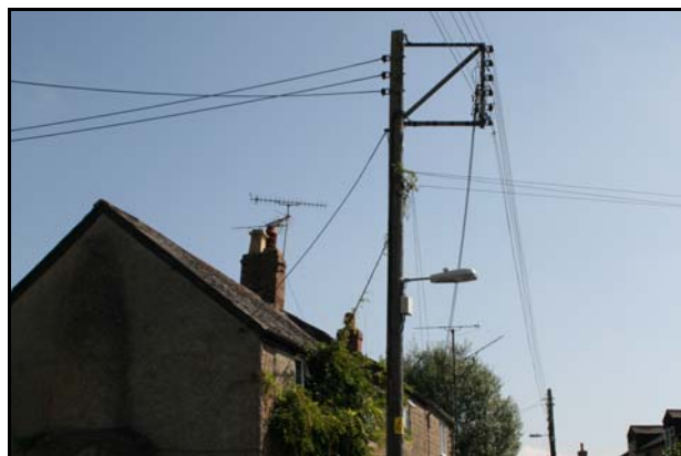
Poles and wires in Rose Lane
